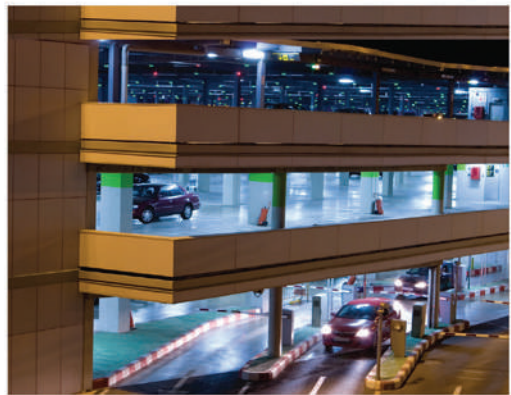
9 level podium parking
